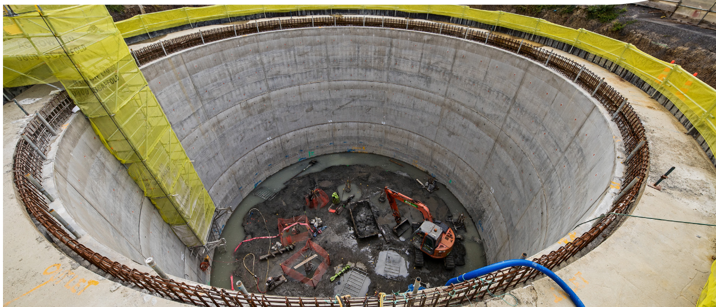
Concrete storage tank 12 metres into the ground.
